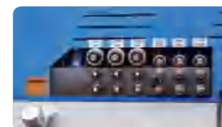
Hydraulic system testing
